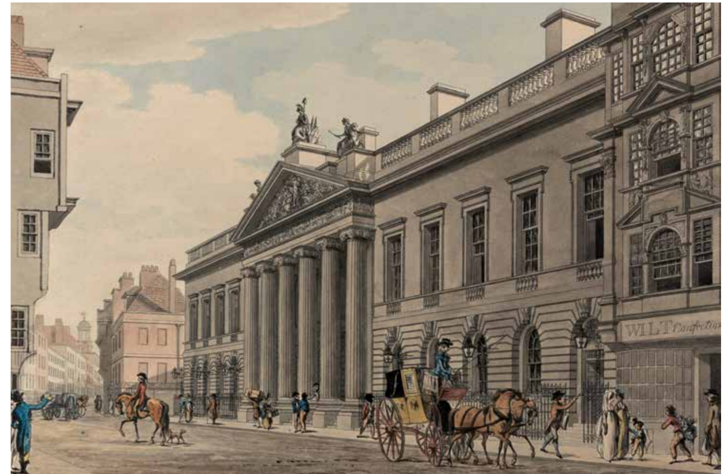
The seat of power: Head Office of East India Company on Leadenhall Street, London
