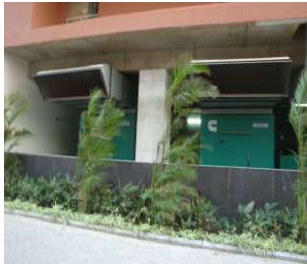
DIESEL GENERATOR SET WITH ACOUSTIC ENCLOSURES
