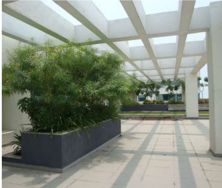
HIGH ALBIDO PAINT HAS BEEN APPLIED AND ROOF TOP GARDEN
